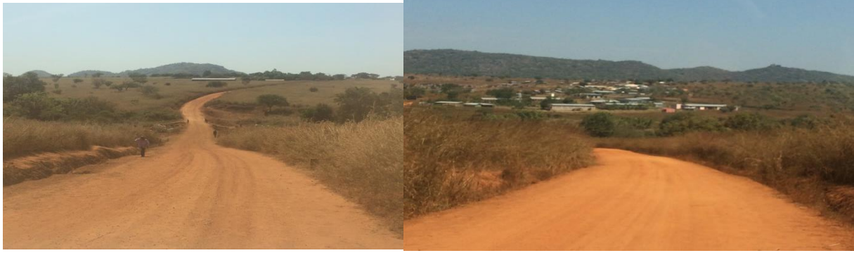
Fig 26:- Road from ARRA Office Compound to Community School in Tsore Refugee Camp.
