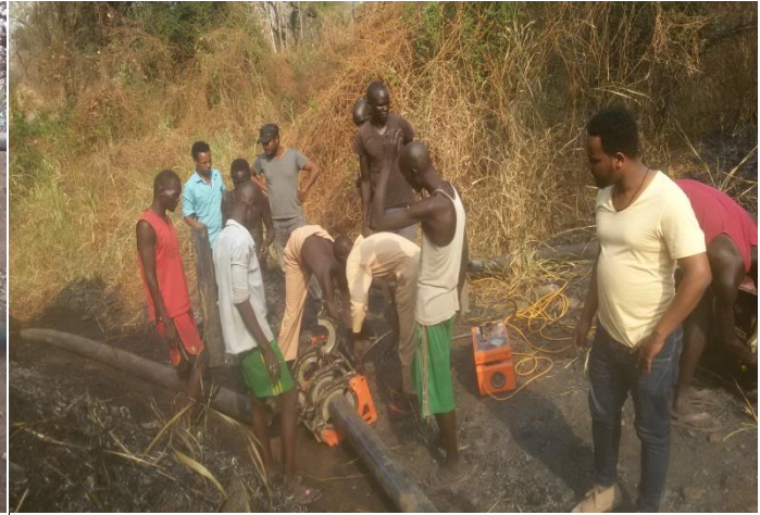
Fig 4 :-During Pipeline Maintenance In Jewi
