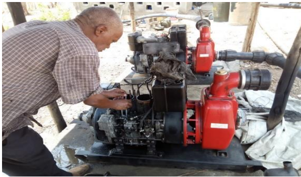
Fig 5:- During pump and generator maintenance Jewi
