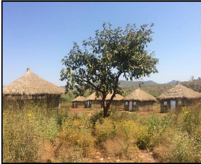
Fig17:- Transitional Shelter (Tukul) @ Tsore Refugee Camp (Assosa)
