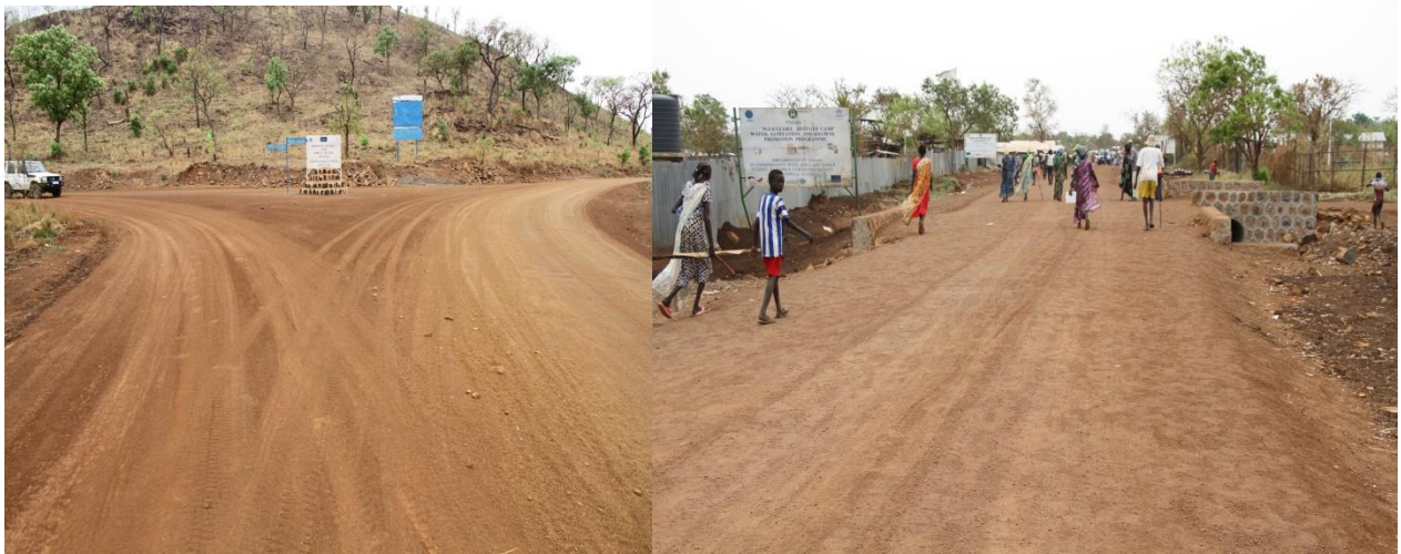
Fig 21:- Access Road Maintenance in Gambella Operation
