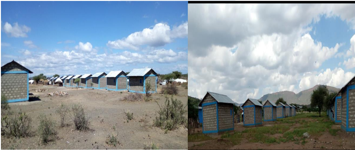
Fig 20:- Completed HCB Improved Transitional shelters in Dillo and Megado Refugee camps
