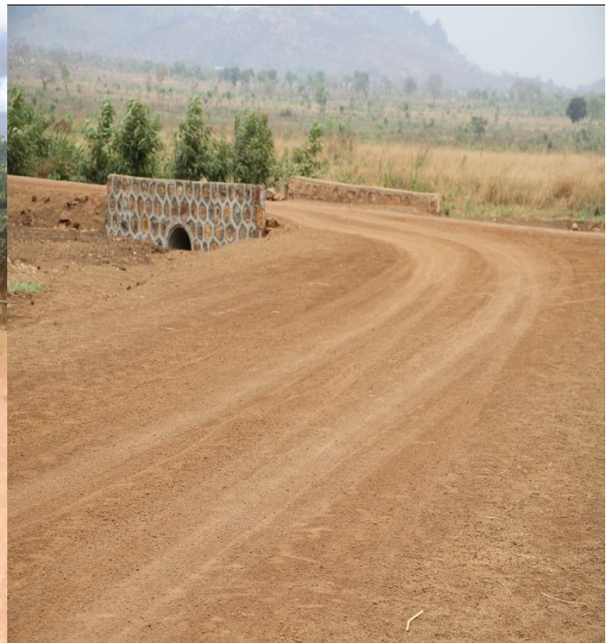
Access road maintenance to Kule refugee camp UNHCR[2018]
