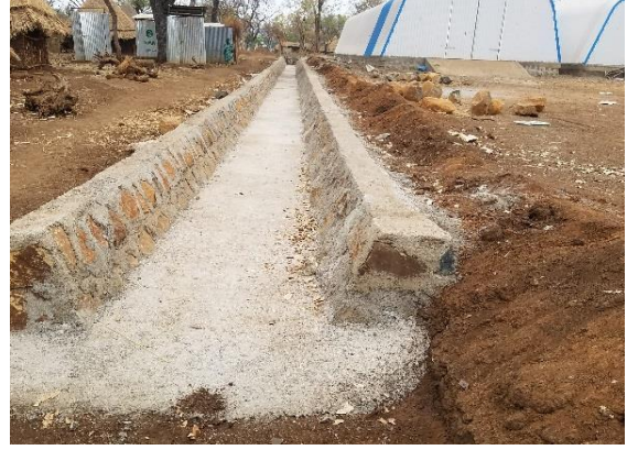
Fig 29 and 30:- Completed platform (Left) & Drainage Ditch construction (Right) at Nguenyiel Refugee camp, Gambella
